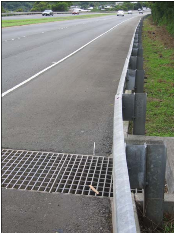
Storm Drain along Kalanianaʻole Highway
